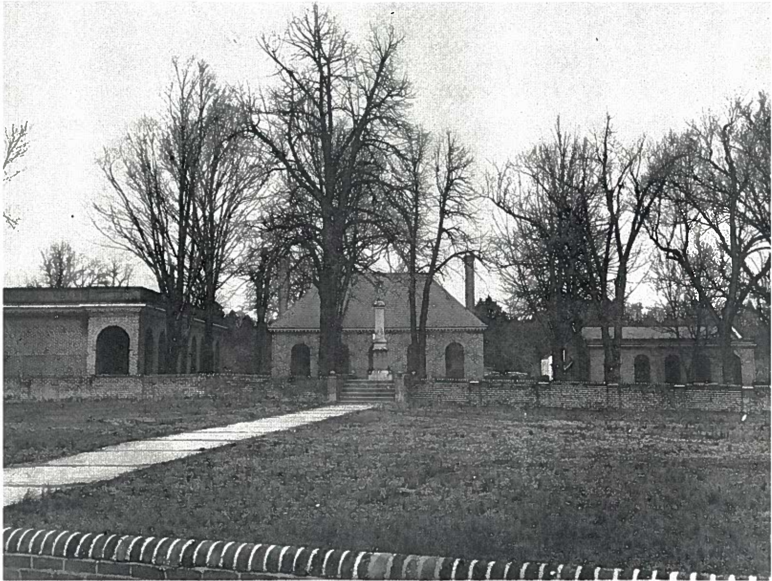
King William Courthouse and offices as they are today.
